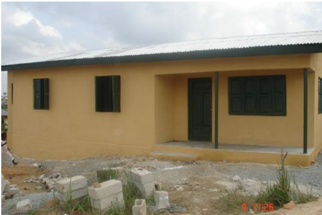
New Structure Tamba Ngaujah C 116 5 Bedrooms + 2 service space
